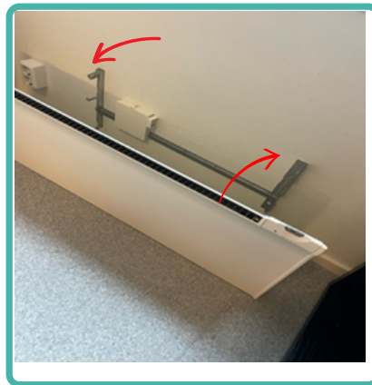
Detach wallheater and clean front and backside
