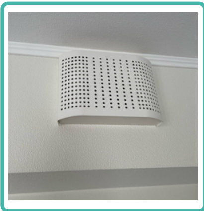
Remove dust from ventilation grid
