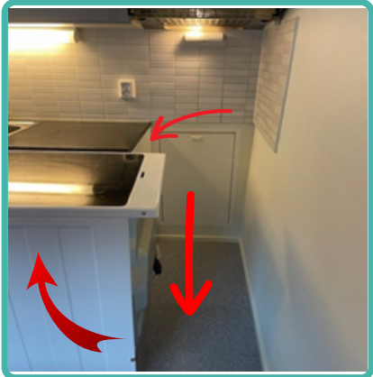
Clean the floor, floormouldings behind and the sides
