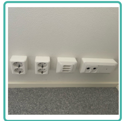
Outlets and sockets : remove dust and stains
